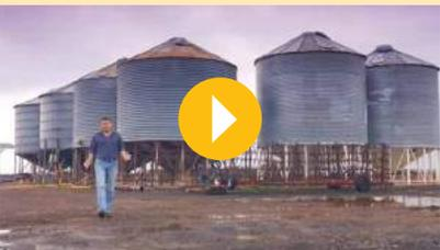
may not have been gas-tight from the day they were constructed. However, even a silo that was gas-tight to the standard on construction will deteriorate over time, so it needs annual maintenance to remain gas-tight.
