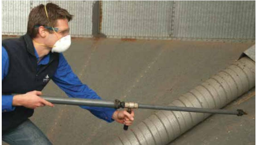
**Photo 7:** Clean silos, including the silo wall, with air or water to provide a residue-free surface to apply structural treatments.
