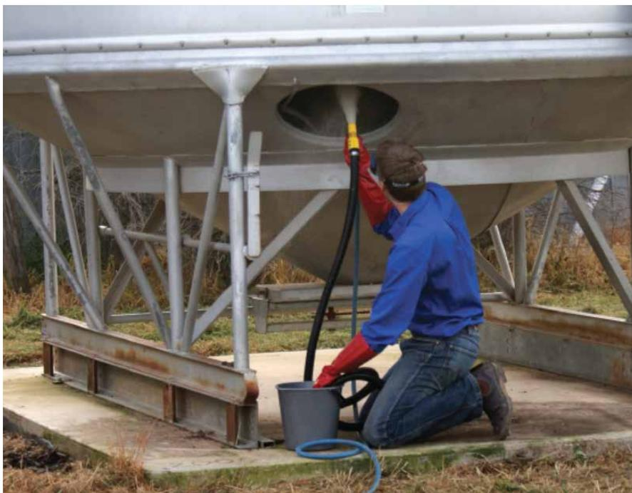
**Photo 9:** A blower–vacuum gun such as the Venturi gun is the best applicator for inert dusts. Aim for an event coat of diatomaceous earth across the roof, walls and base.
