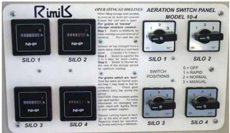
**Photo 12:** Automatic aeration controllers are the most effective way to cool grain and are designed to manage many storages from a central control unit.
